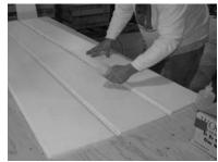
5) Lay 3 panels flat and apply adhesive to center joints. (Polyurethane glue is recommended. Follow manufacturer's instructions.)
