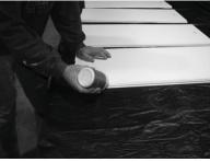
3) Apply polyurethane glue to both edges of ONE PANEL only.
