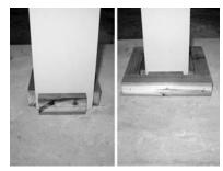
2) Install blocking around load bearing post (use pressure treated lumber.) Final width of blocking must be same width as inside of column.
