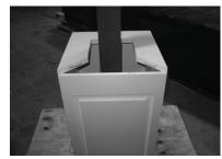
9) Note: top platform usually extends beyond top of shaft section (not shown in photo). Mouldings are applied under the top platform. Assemble top platform on top of shaft. Glue mitered edges, and attach with pin-nails. (Pyramid caps do not use top platform.)
