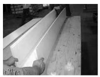
6) Assemble three panels, using E-Z Lock joints.
