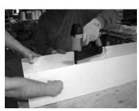
7) Using finish nails, assemble three panels together. Observe EZ-Lock diagram on reverse to determine correct nail placement.
