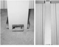
3) If desired, optional blocking (not provided) may be installed around post to center wrap. This is especially helpful when wrapping round or odd sized supports.
