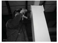
15) Option 1: Attach cap to soffit with construction adhesive and toenail to soffit. DO NOT ATTACH cap to column shaft if the cap is flush with soffit (to allow expansion).\*
