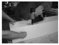
7) Using finish nails, assemble three panels together. Observe EZ-Lock diagram on reverse to determine correct nail placement.
