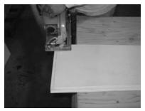
2) Trim shaft pieces to 2½" shorter than opening—2" for cap/base, ½" for expansion (½" if not using cap and base—each part is 1" thick.) Always trim from bottom ONLY-top is marked.
