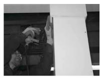
16) Option 2: Leave <sup>1</sup>/<sub>4</sub>" expansion room above cap, and pin-nail the cap to the column. Be sure the pin-nails DO NOT reach the blocking inside!\*
