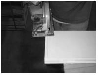
2) PVC expands and contracts with temperature changes. Trim shaft pieces to 1/2" shorter than opening height (from step 1) to allow for product expansion.
