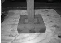
1) Install blocking around load bearing support (typically pressure treated post). Blocking should be made from pressure treated wood, and must be the same size as the inside of the pedestal/newel.
